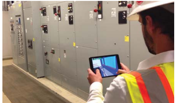
Shane Saltzgeber, project manager for St. Francis Electric, in the substation looking at a 3D Model of the site on an iPad mini. The 3D Model image shows the subsurface conduit and structures underneath the substation floor using BIM 360 Glue's augmented reality capability
